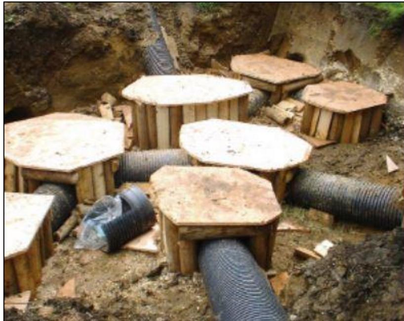
*Figure 5-15 An example of an artificial sett under construction with pipe tunnels and 7 chambers (Extracted from NRA (now TII), 2005b)*
